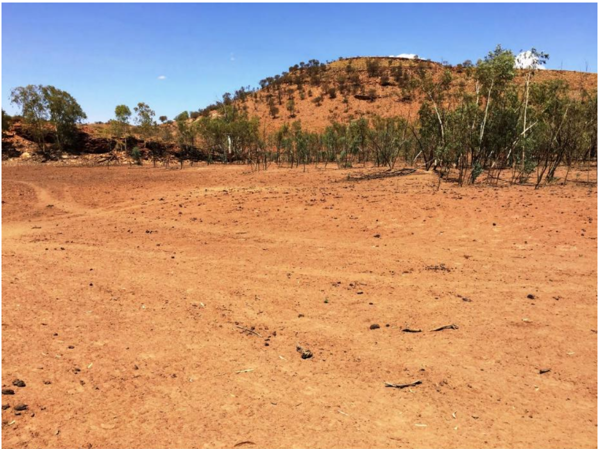
Figure 6: Dam at Jervois before recent rain.
